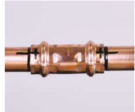
6. Mark the completed joint
