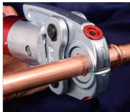
5. Complete the joint with the press tool
