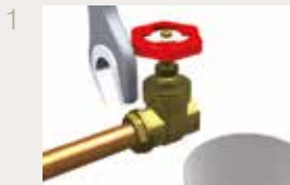
After turning off the water supply undo fitting using a spanner
