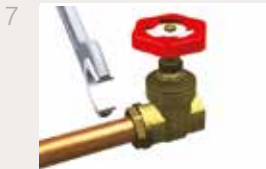
Tighten with a spanner until secure
