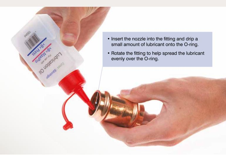
Conex Bänninger Press Fitting Lubricant
