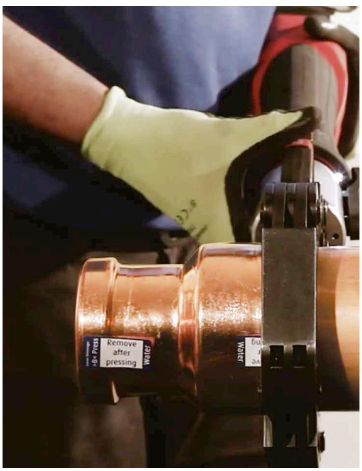
To install >B< Press XL, a press tool, actuator and compatible sized press ring to fit each size fitting is required. When force is exerted through the press tool a permanent joint is made and the fitting cannot be disassembled or reused.
