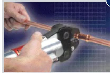
**3** Depress the trigger/button to begin the compression cycle of the tool. This is complete when the mouth of the fitting is fully enclosed by the jaws. Now release the jaws from around the fitting. (For further information refer to tool manufacturer's instructions.)
