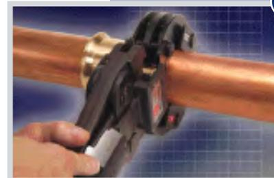
**7** On completion of the pressing operation an audible bleep will be heard; disengage the adaptor by depressing the jaw levers and remove the collar from the fitting. See below for 108mm fitting.
